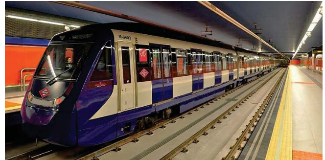
Fig. 2. Train under test
