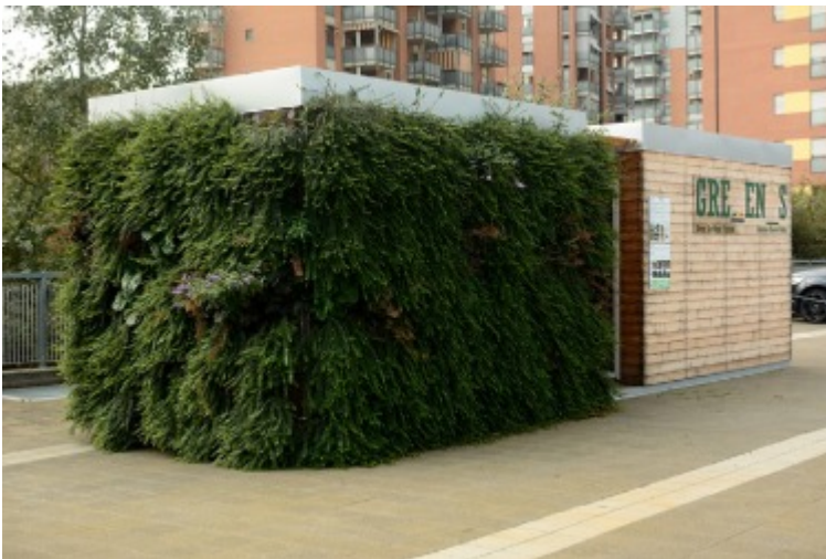
Fig. 21. Demonstration mock-up, 1 year after plantation (Environment Park, Turin, Italy).
