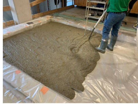
Figure 3. Application of the EPS thermal layer
