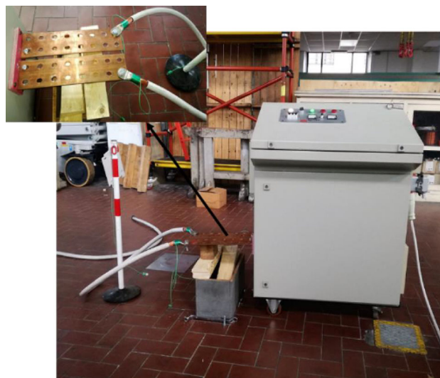
Fig. 9 View of the heating setup with the OS.A.T current generator (right side) supplying, through two copper bars, the cable headed with the two crimped lugs whose R_{crimp} has to be measured
